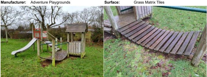
Finding: The bridge is making contact with the surface
