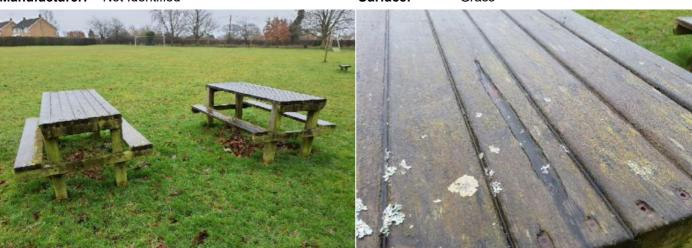
**Finding:** There are areas or parts of the timber on the structure that have rotted
