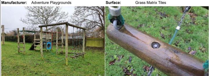
Finding: There is/are bolt cap covers missing or damaged Action: Replace missing or damaged bolt cap covers on the item
