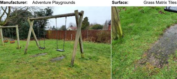
**Finding:** The grass mats are silted up and the soil is compacted; this may have an effect on the impact absorbing properties of the surface. Consideration should be given to HIC testing the surface to verify impact attenuating properties ( https://playinspections.co.uk/inspectionservices/safety-surface-testing/ )
